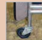
Replaced broken casters
